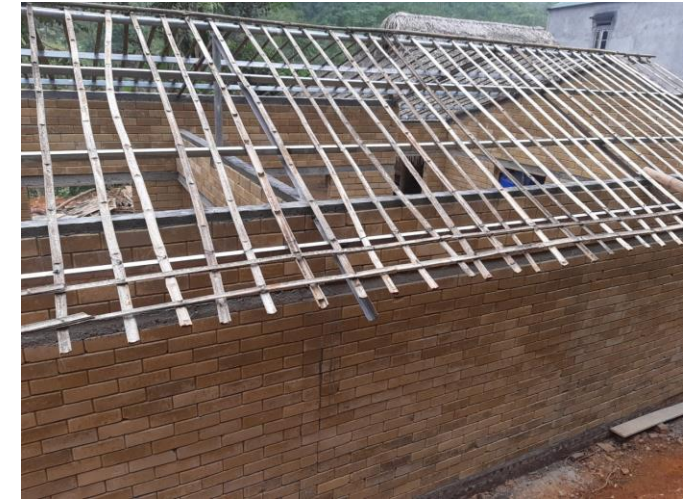
Bamboo supports the palm roof
