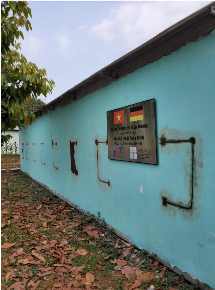
On the exterior face of the wall
