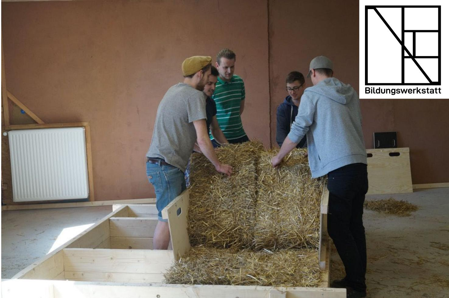
The density from the straw building guideline is what matters: Simple prefab technique for modules suitable for passive houses, install the last 4 straw bales at
