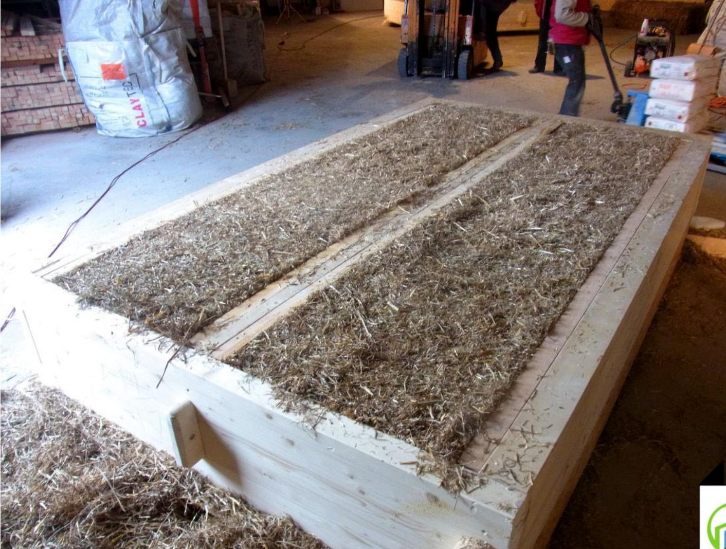
NZNB, Prefabrication of the elements took place directly in the adjacent Workshop by <https://Baustroh.de> GmbH Baudokumentation:
