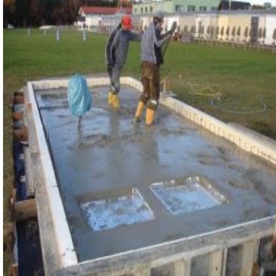
Example Foam Glass Gravel Load bearing insulation under ground slabs
