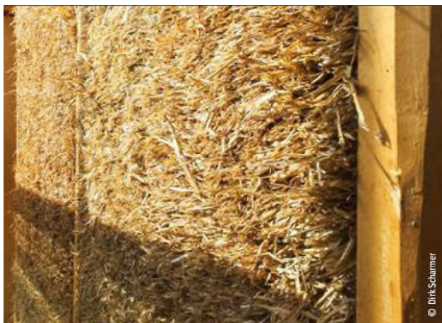
Figure 13: Photo of a wall with straw insulation [ 6 ].
