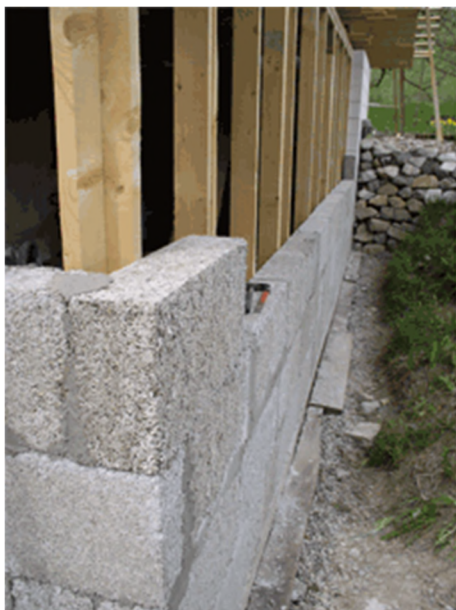
Figure 2: Wall with hemp blocks, photo from [ 7 ].
