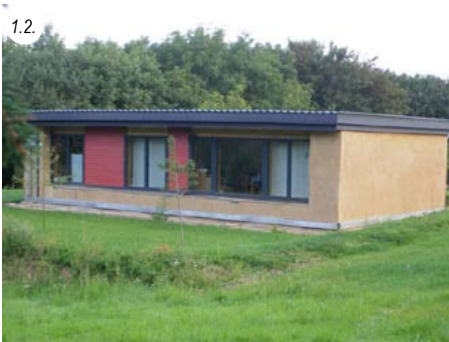
Finished, walls load-bearing with large bales
