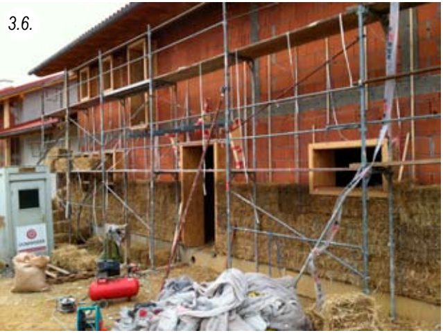
New brick building with a straw façade doveled on bricks
