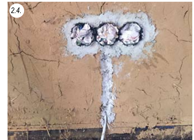
Electrical sockets mounted in rough clay plaster with rapid cement, cables preferably damp-proof cables instead of pull-in wires (tightness)
