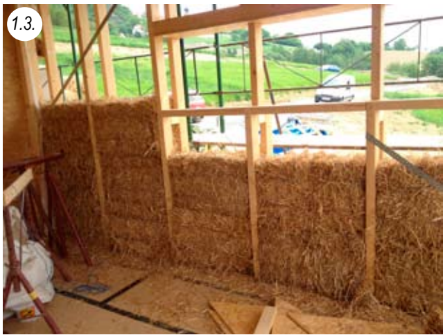
Filling goes quickly if the bales fit
