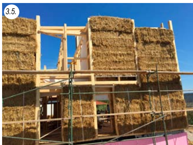
In the case of large bales, only whole and half bales should be included in the planning concept (with a theoretical length+ 5cm)
