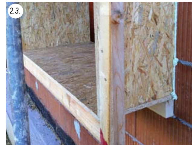
Window box here up to the inside edge of the masonry, continuously and extensively glued to the masonry with a smoothline
