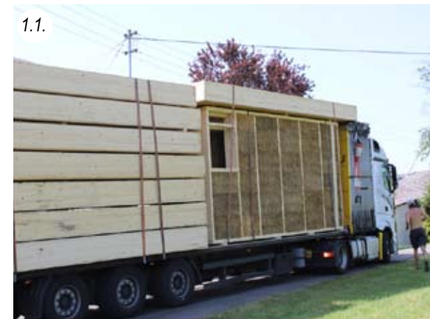
Delivering the prefab elements to the site
