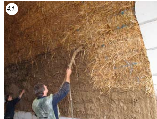
Vault finished with small bales - clay plaster is applied inside
