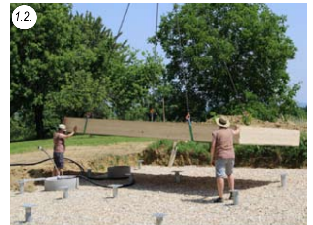
Positioning the floor modules on the screw foundation
