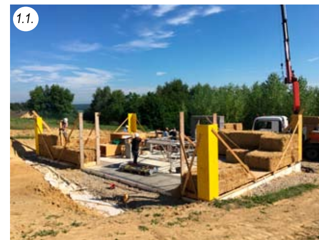
1.1. Floor slab in concrete insulated with Liapor Ground. Straw bales are moved with a crane
