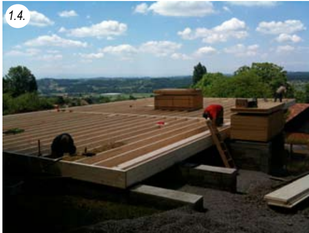
Large base plate protruding into the valley before filling
