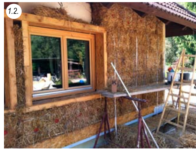
Straw bale facade grows constantly up to the sloping roof
