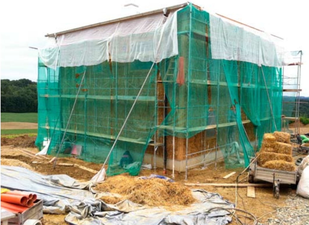
Facade suspended during construction. Protected at the top with plastic tarpaulin and with facade mesh on side.
