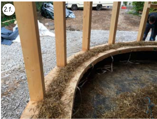
8/16 timber posts, here on the outside so that the bales do not press outwards despite the curve
