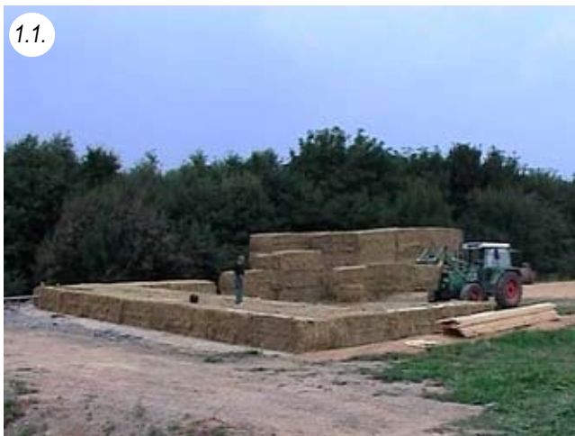
Concrete-free floor slab with BigBales in Germany
