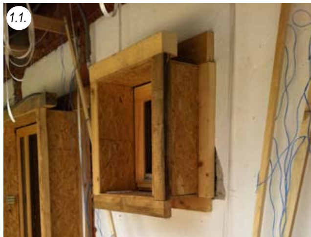
Window and door boxes installed in the old building
