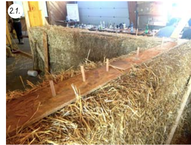
OSB intermediate layer after 4 bales, fixed with wooden nails Better: (hard)-plywood, 20-25cm x 10-12mm
