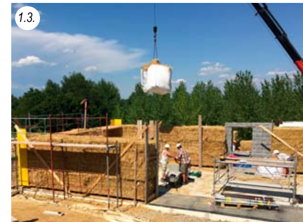
1.3. Loose straw in the BigBag is used to plug the joints
