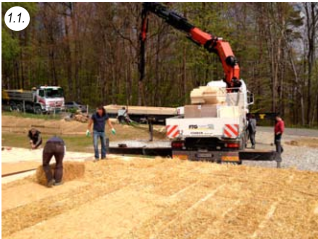
Bales are installed lengthwise between the 8/36 laminated beams and the strings are cut to close any joints
