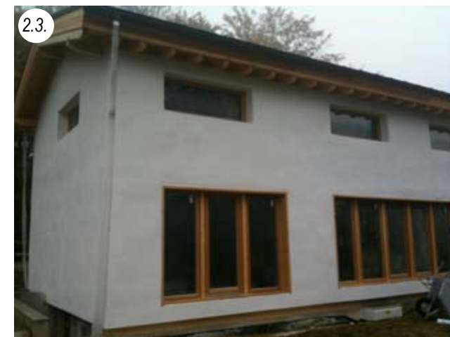
Timber frame+ straw bale facade NUA: 180 m 2 Built: 2009
