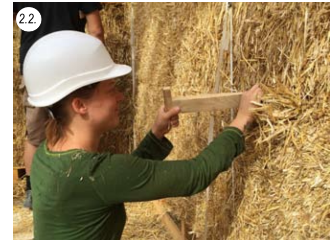
Tool for stuffing loose straw into gaps
