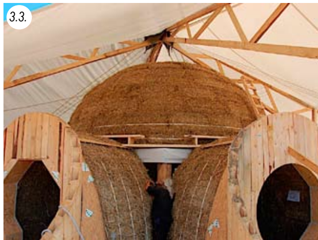
During construction, individual barrel vaults clearly visible
