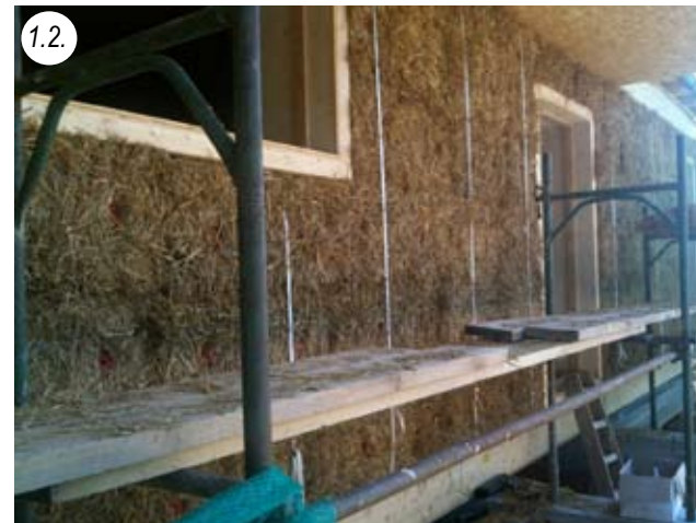
1.2. Straps tight, red dowel plates visible, 2 per bale, all timber construction is flush with bales, 36 cm of OSB
