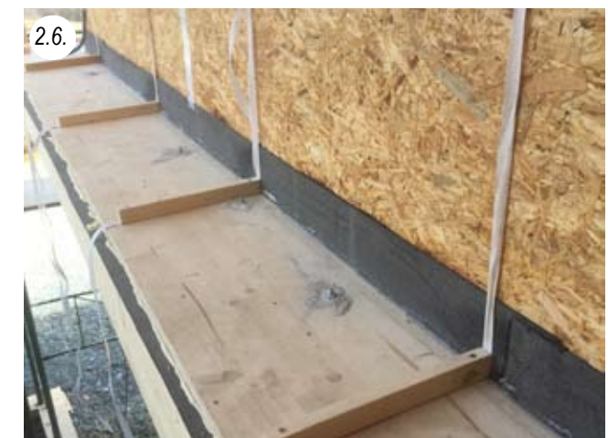
2.6. Bale support (e.g. 30 mm 3-layer board) mounts the strips, with which the tension belts are fixed, clearly visible
