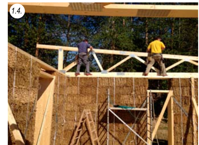
Prefabricated nail trusses are assembled
