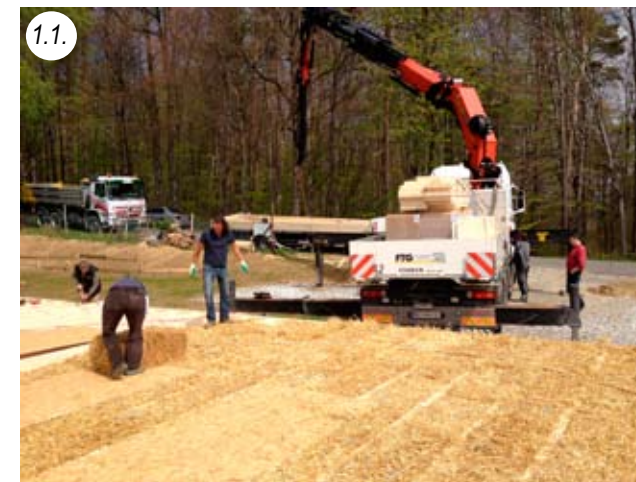
Filling the base plate with straw bales
