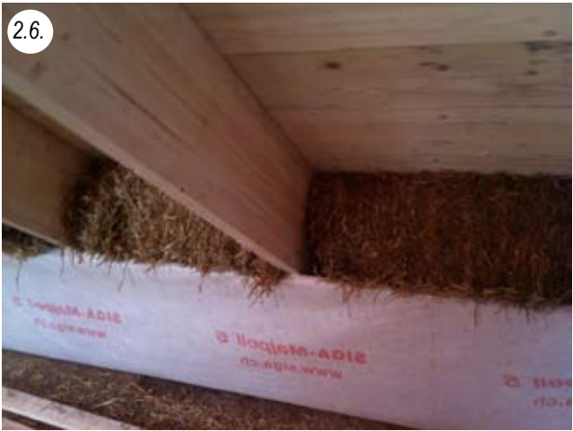
Installed from the inside, following with boards and foil
