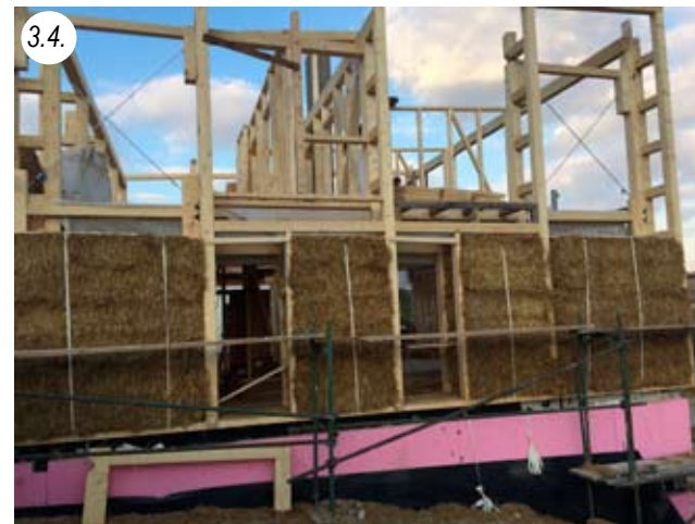
Ground floor precompressed and ready after one day
