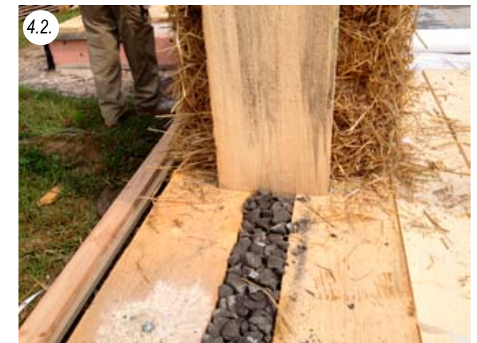
Base with foam glass fill in the „condensate pocket“
