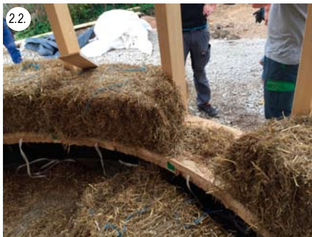
Bales are slightly curved before attaching
