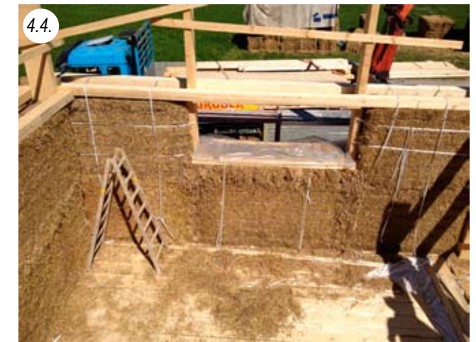
Window openings are based on the bale size
