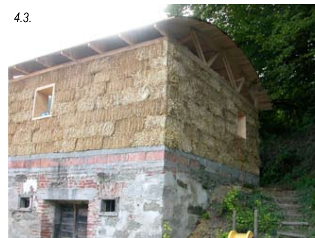
First load-bearing building approved in Austria Client + straw bale construction: Virko Kade Built: 2004
