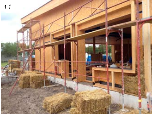
1.1. Starting with counting the straw bales, -many windows require a lot of time resizing the bales
