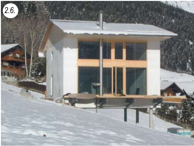
Load-bearing with BigBales, Switzerland, Arch. Werner Schmidt
