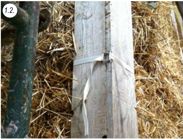
Halfway up the wall, the corner guide is connected to wall underneath so the bales don't push it out
