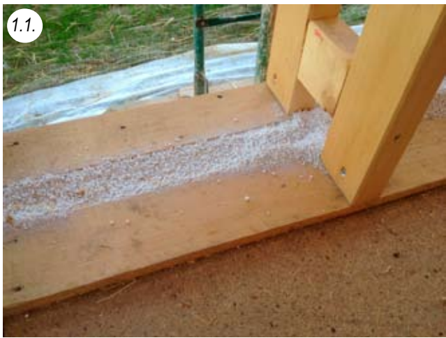
Pedestal with perlite filling, ready for the first bales
