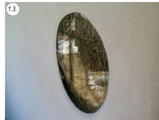
„Truth window“ plastered into a straw facade
