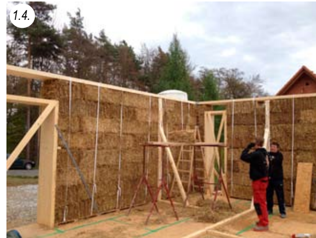
Wall with ring beam ready for the rafters
