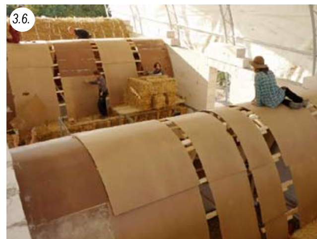
The formwork
