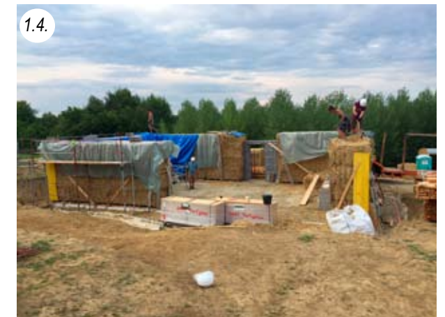
1.4. Covering the top of the wall is sufficient in light rain
