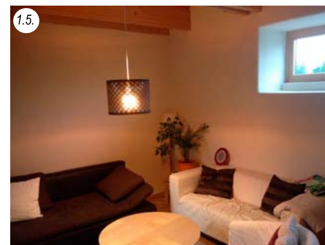
Clay plaster on large bales inside, surface painted with white clay
