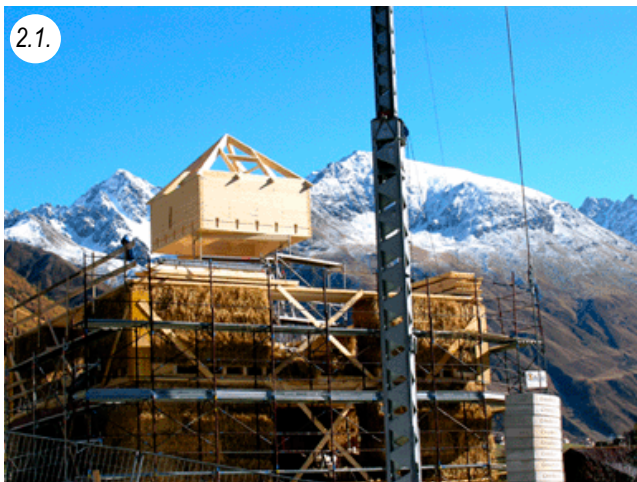
Load-bearing with big bales - Arch. Werner Schmidt/Switzerland
