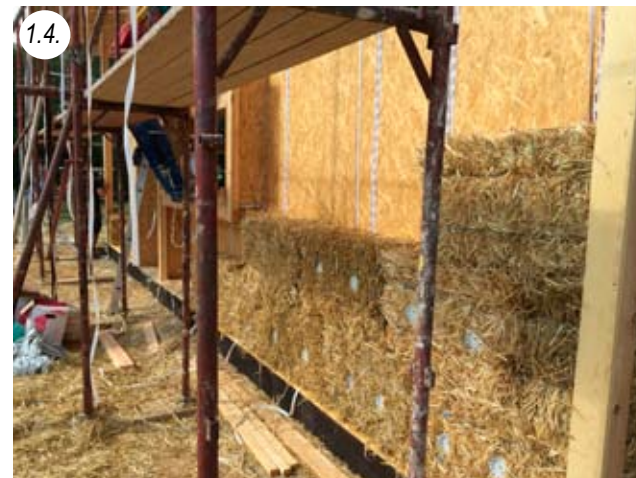
1.4. Corner guides made of 2 boards screwed on each other at right angles, helps with bale assembly and gives nicer plaster edges
