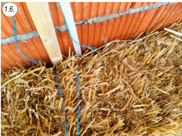
Installation variant with strips and string (for old brick buildings often better than with dowels due to poor brick quality)
