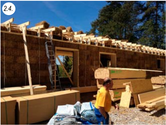
Bales can be brought in from the outside or distributed between the rafters and separated
