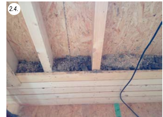
2.4. Filling in the installation level
