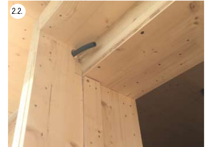
2.2. Detail of window frame with connection for venetian blind motor
