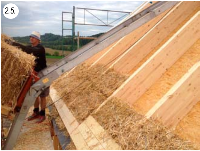
Saddle roof with insulated roof space, inserted from the outside
