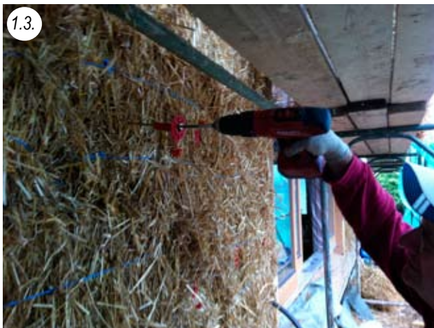
1.3. Mounting the bales with insulation plugs /dowels
