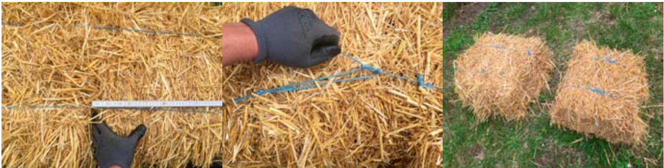
Measure bales and form joints with your hands, then untie cords Wrap cords around the newly formed bale, press and knot (pulley block) Finished bales
