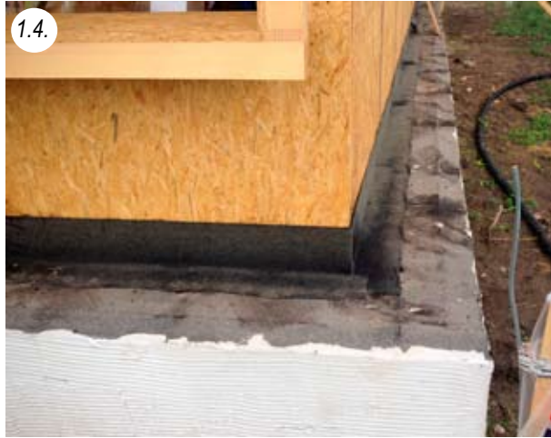
Base glued with bitumen before 3-layer board is mounted
