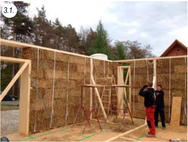
Load-bearing with small bales, lying flat
