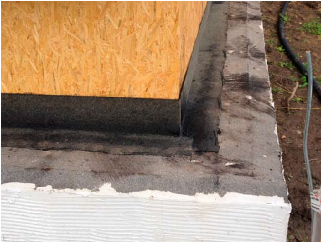
Perimeter insulation (XPS) neatly sealed base. Ready to receive a 3-layer panel and the first bales of straw.
