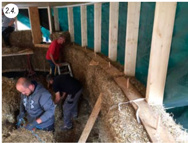
An intermediate layer, fixed with wooden nails, is tied to the posts for a better bond
