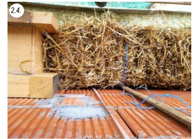
Window box and battens with bale string for later fixing the bamboo sticks, no dowels here
