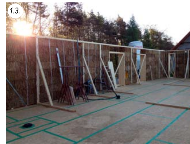
After 2.5 days of straw construction, the outer walls are in place and the roof truss can be installed
