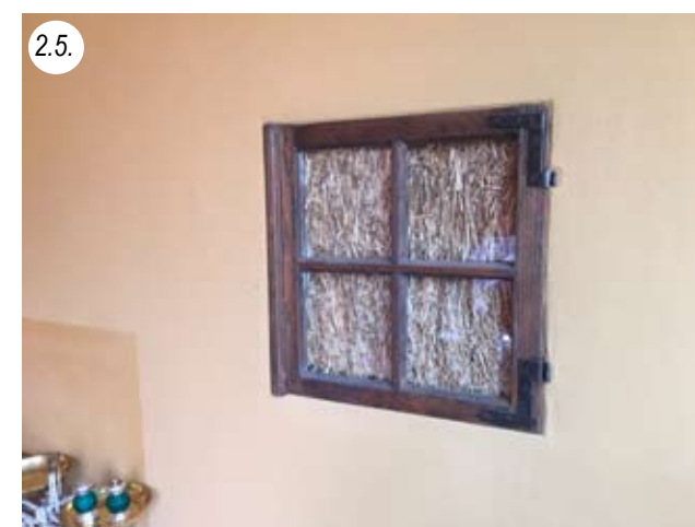
„Truth window“ built into the clay layer inside
