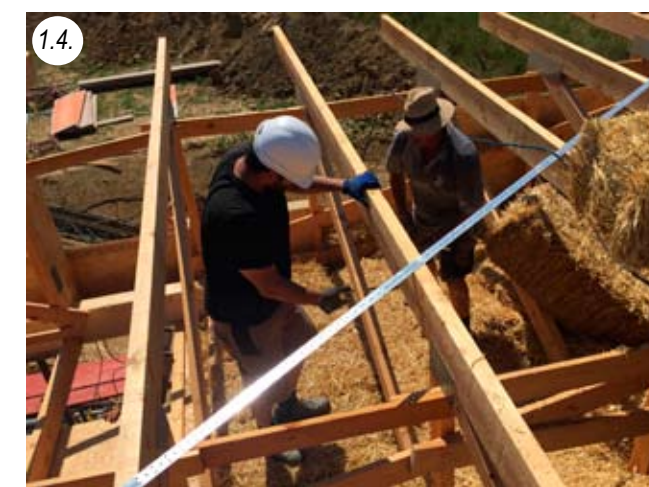
1.4. 2 layers of small bales are brought in from above, strings cut later
