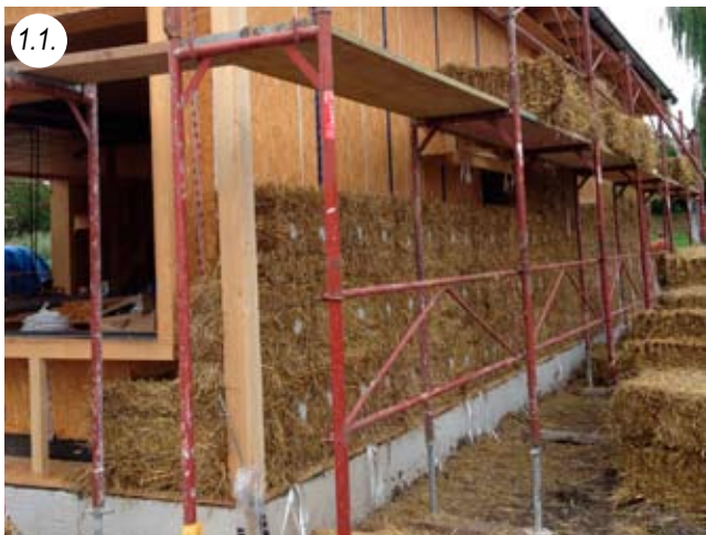
Corner guide: choose orientation of the bales very carefully here
