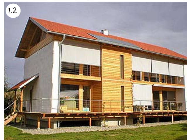
Timber frame+ straw facade NUA: 220 m 2 Built: 2006
