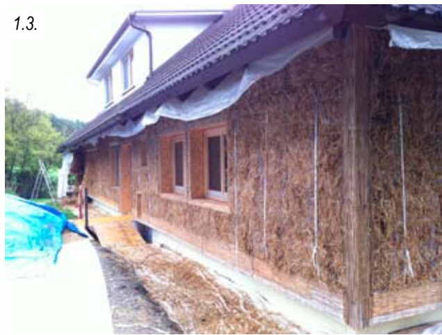
Ready for plastering, reed stucco clearly visible on corner brackets / guides and window boxes
