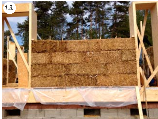
After 4 out of a maximum of 8 layers, assembly of the tension system
