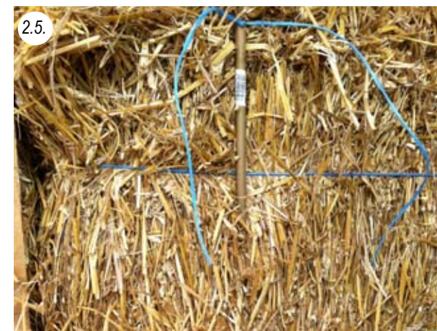
Bamboo stick visible, but disappears almost completely in the bale
