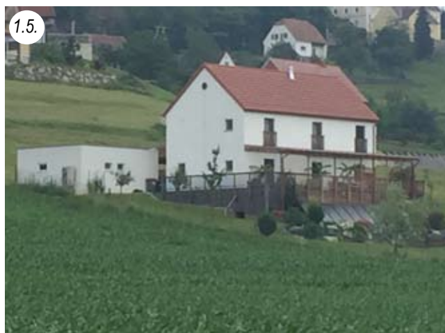
Ladder system, straw plastered on both sides NUA: 180 m 2 Built: 2014
