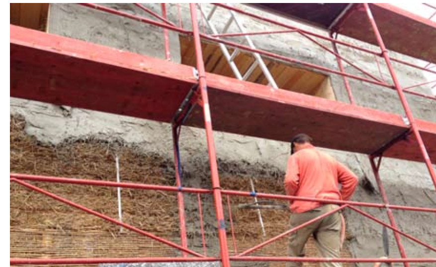
The first layer of lime plaster is sprayed onto the straw bale wall
