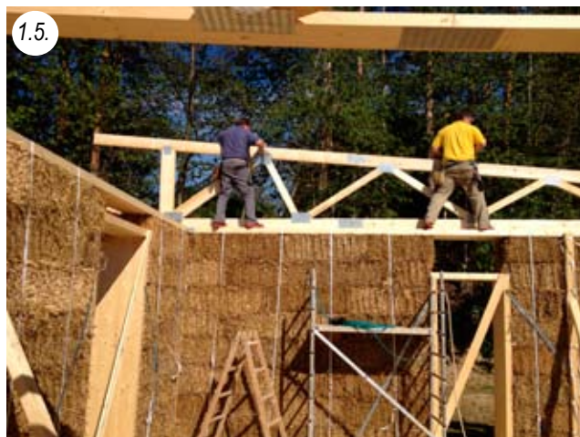
Rafters here as a nail truss with low weight and quick assembly
