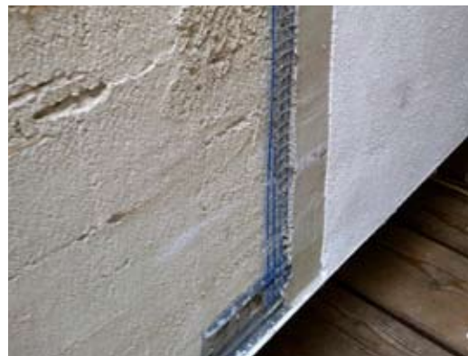
Lime plaster structure with drip edge, here base plate in wood plastered on the front, the plastered straw bale wall already begins in the upper area
