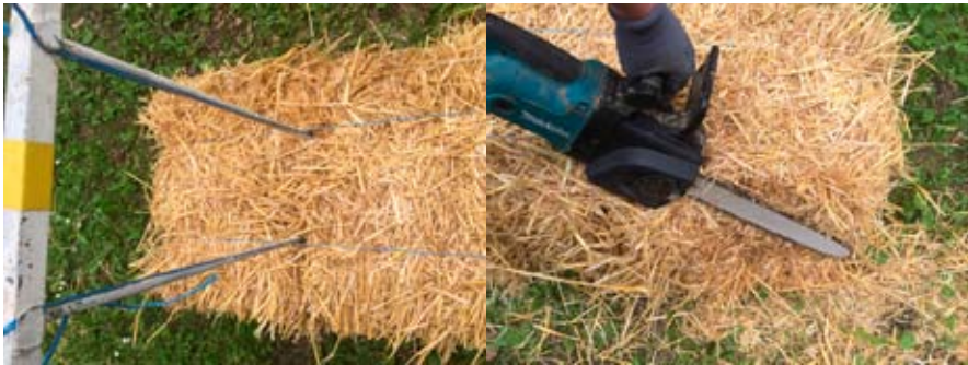
Pierce at a measured point. Turn the bale and tie it again Longitudinal cuts with chainsaw or alligator.
