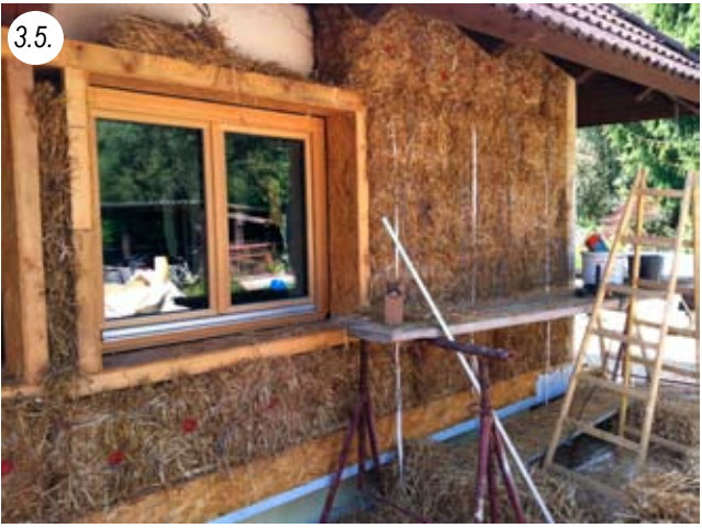
Old brick building, straw facade in front, bales mounted on edge
