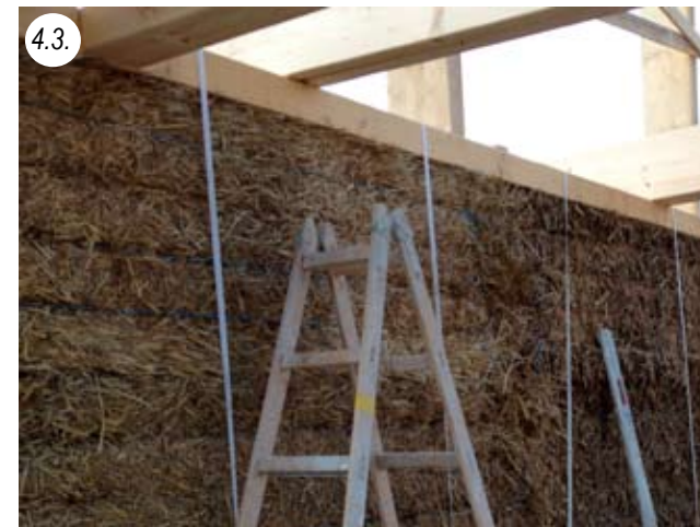
Intermediate ceiling lies on the straw bales, only after setting bolted to posts and then continue to built on the upper floor
