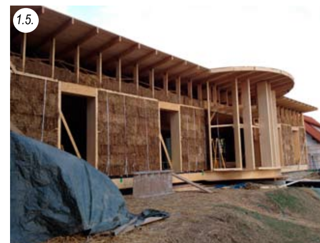
The roof skin is rain tight, the roof truss is insulated, the settlement is complete, only a few plaster preparations are left
