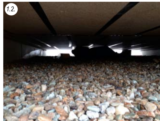
Drained gravel bed underneath wooden floor plate
