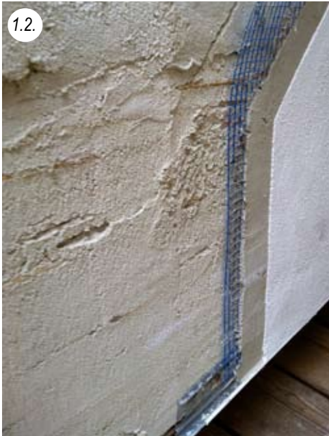
Socket profile with drip edge. Variant in metal. If there is a high proportion of splashing water, the lower edge must be well connected/glued with bitumen. Clearly visible: rough plaster, mesh plaster, fine plaster.
