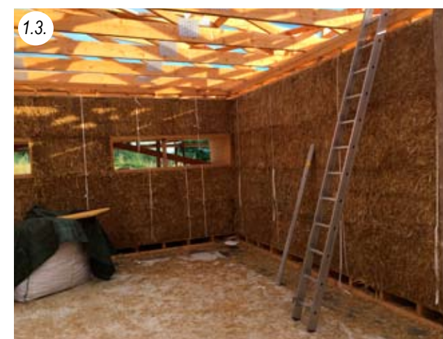
1.3. Completely assembled, ready for the formwork onto ceiling
