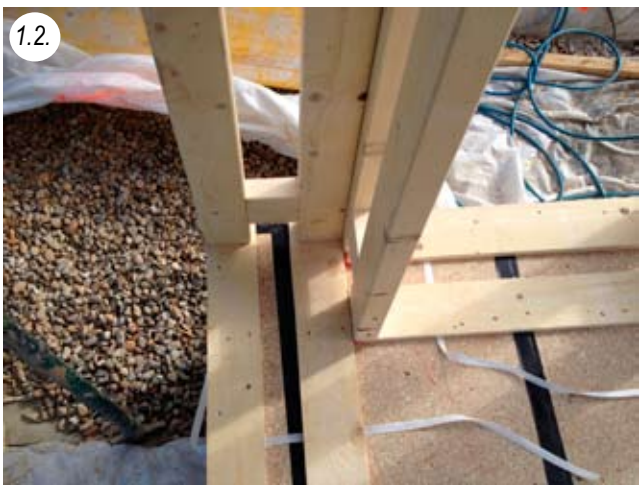
Plinth detail in the corner of the building, with tension belts visible
