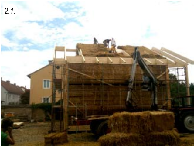
Bales are lifted onto the roof with a crane
