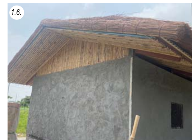
First layers of plaster finished
