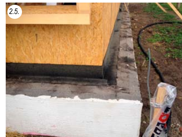
2.5. Base sealing before installation of the bale support, here concrete slab insulated with Liapor and XPS on the front side
