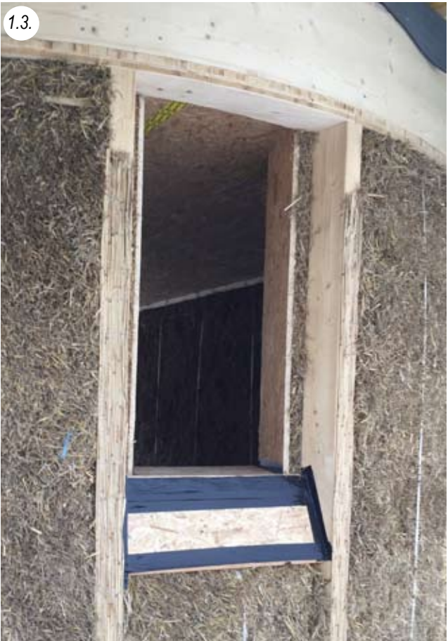
Window frame for variant without window sill, before scratch render
