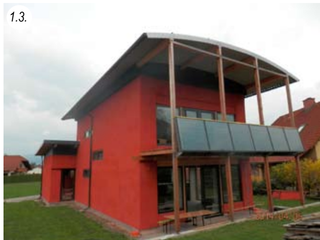
BigBales with ladder system, partially load-bearing, plastered on both sides NUA: 170 m 2 Built: 2012
