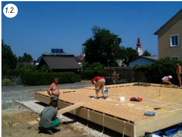
Finished floor slab with at least 30 cm ventilation and gravel bed, the bonding of the slab joints is also clearly visible
