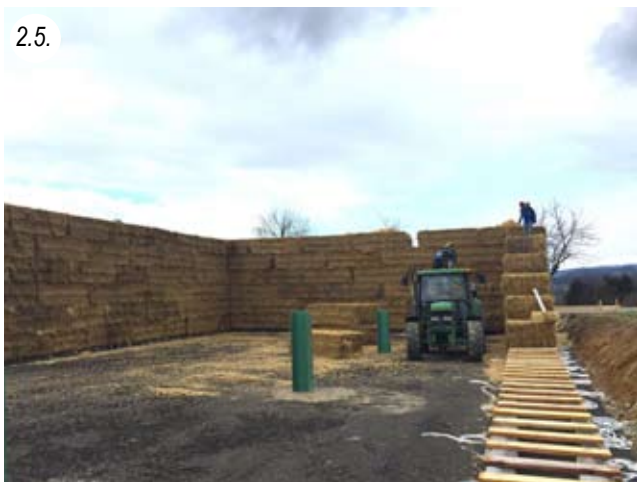
Load-bearing machine hall with big bales, for company Sonnen-Klee (A) -Project of the author
