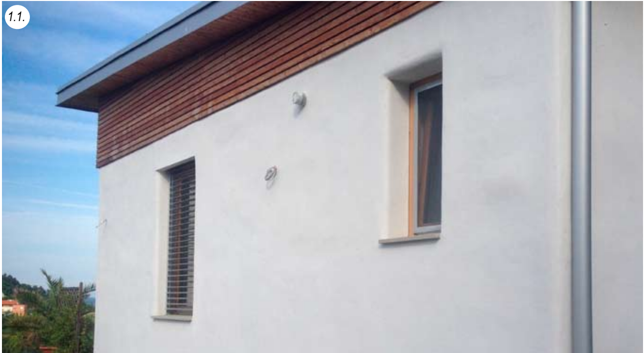
Windows with and without external blinds, window sill and plaster finished
