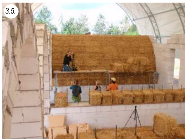
Load-bearing barrel vault in Wangelin/ Germany
