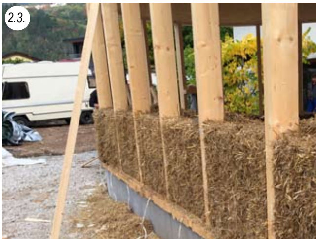
With one post, inside or outside, the bale is usually installed lying flat
