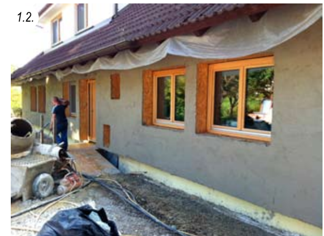
2x scratch coat of plaster, straw is no longer visible, on the left plastering machine for lime and clay plaster
