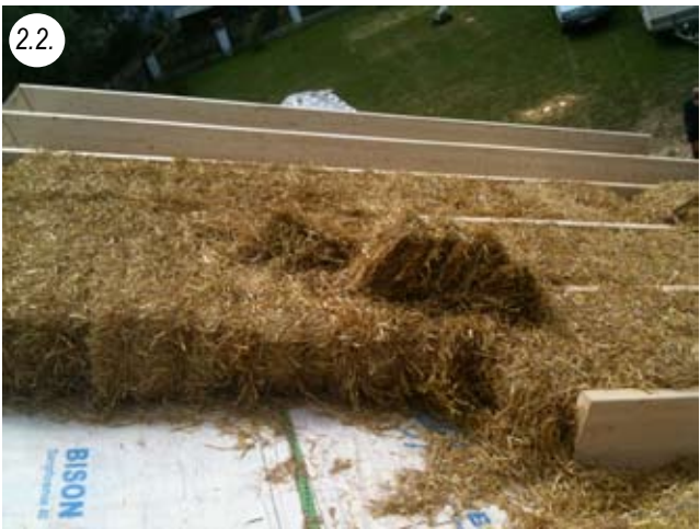
Cold roof structure mounted floating on the straw bales, with Boards directly on the bales, then foil + battens
