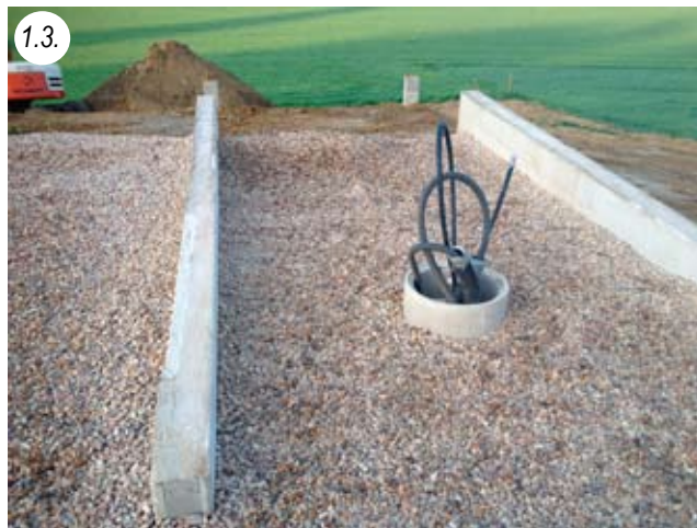
Installations combined in a concrete shaft and led into the floor slab, later all cavities filled with perlite
