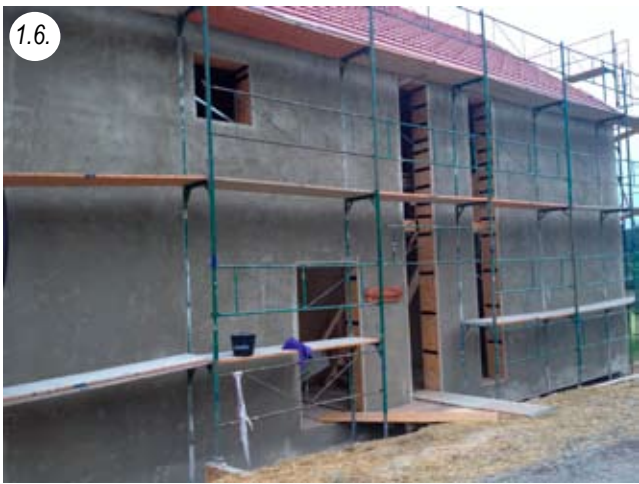
After the first layer of plaster
