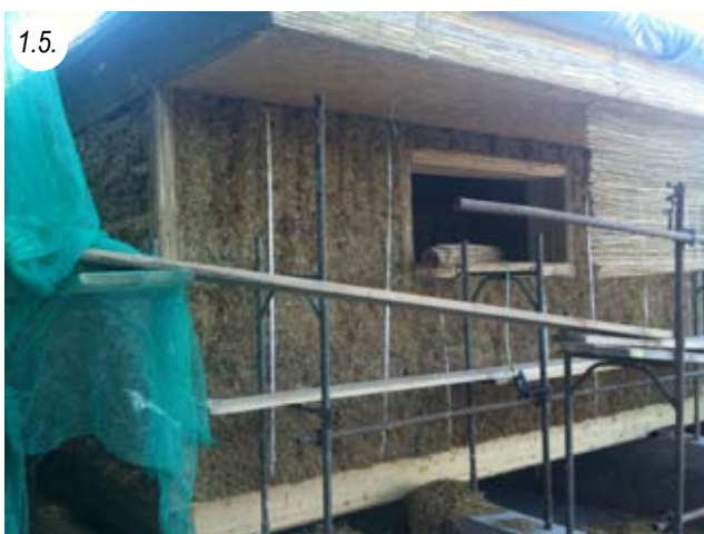
1.5. All plastered wooden surfaces are previously covered with reed mats, here the eaves in process
