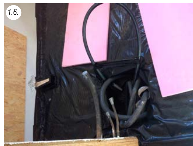
Entire floor in the technical room with pond liner, including elevation the walls, in the event of a pipe break, drainage into the concrete shaft and further into the gravel bed is possible
