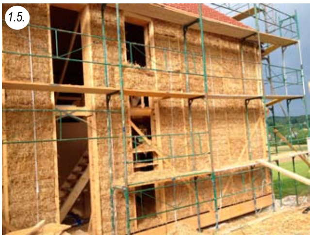
Straw insulation going through both floors without interruption
