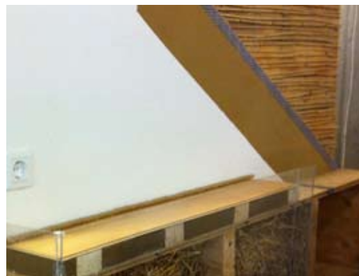
Clay plaster construction with reed mats on wooden surface, e.g. for partition walls or construction with an installation level
