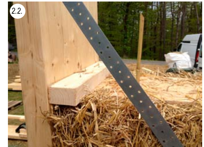
OSB tension system mounted on the window frame
