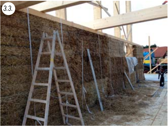
Hybrid system, large bales on edge, partially load-bearing
