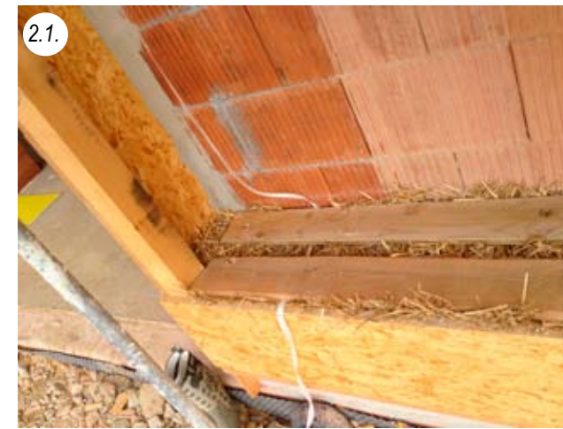
Base box filled with straw, belts threaded, ready for the first bales
