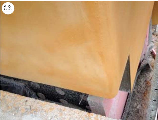
Socket profile already plastered, here in plastic, cut and bent round
