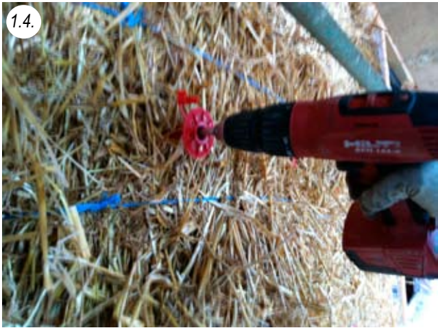
2 dowels per bale, each at 1/4 and 3/4 in bale length, in the middle, have proven to be sufficient in practice, although not certified!
