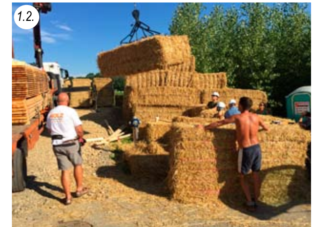
1.2. With big bales, the grapple must work well
