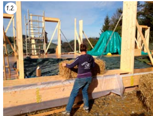
The first bales are positioned
