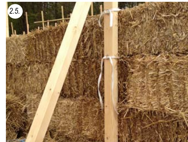
Timber posts for partition walls are „sewn“ with straw bale wall
