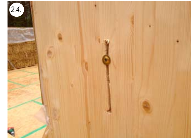
Long hole (slot) to follow settling and still be under tension
