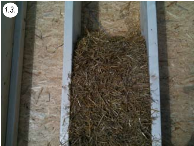
Intermediate size corresponds to the bale width, here 50cm
