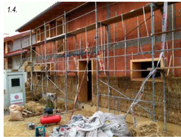
New brick building planned for straw bales, base was done with a row of formwork blocks with intermediate insulation on the outside
