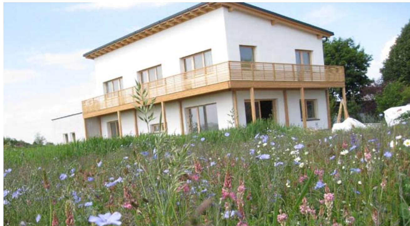
Lime plaster finished, here on directly applied on a straw bale façade, wall structure with installation level
