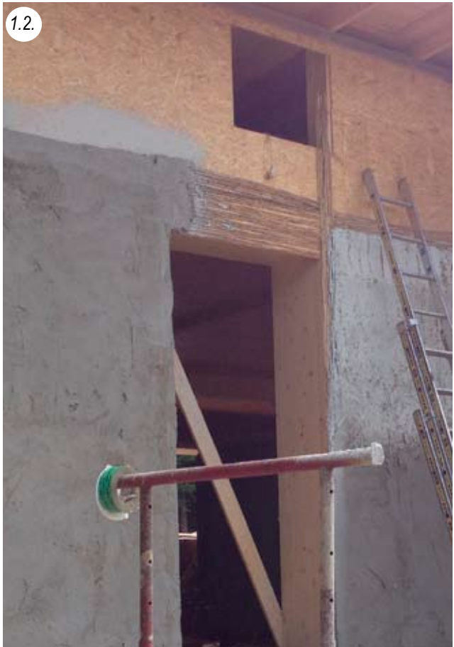
Window frame with rough plaster only on the front side, reed mats can still be seen clearly on the box for the venetian blind
