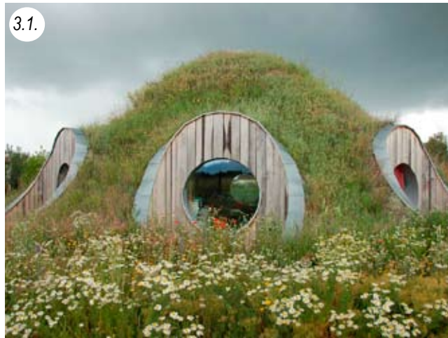
Load-bearing straw dome with grass roof without ventilation. Planning: Gernot Minke, Zuzana Kierulvova / Slovakia
