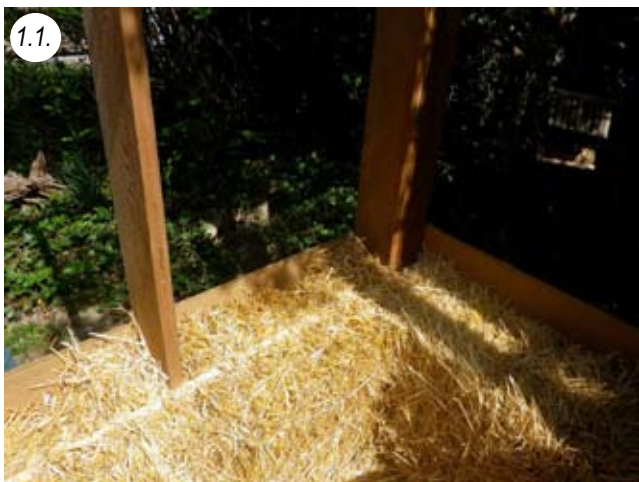
Batten with single post variant and formwork on the outside
