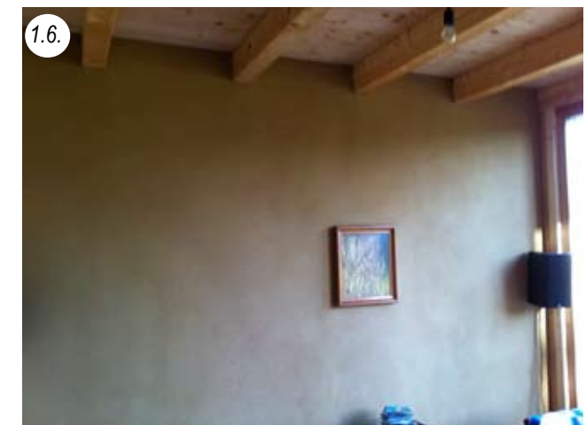
Clay plaster on big bales inside, natural surface
