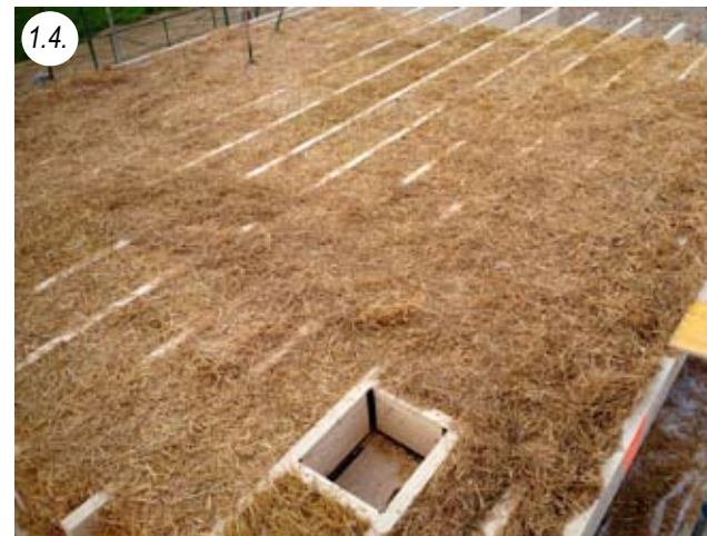
Opening for the passage of all house connections through the straw bale level
