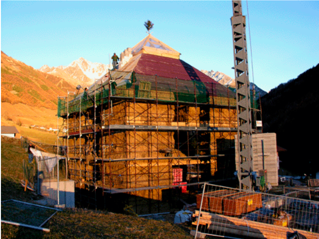
Test object for straw bale construction statics: House Fliri/Switzerland. holiday apartments. 3.5 floors. Only the corners, each consisting of 1.5 large bales, are load-bearing. Large window openings in all 4 directions.
