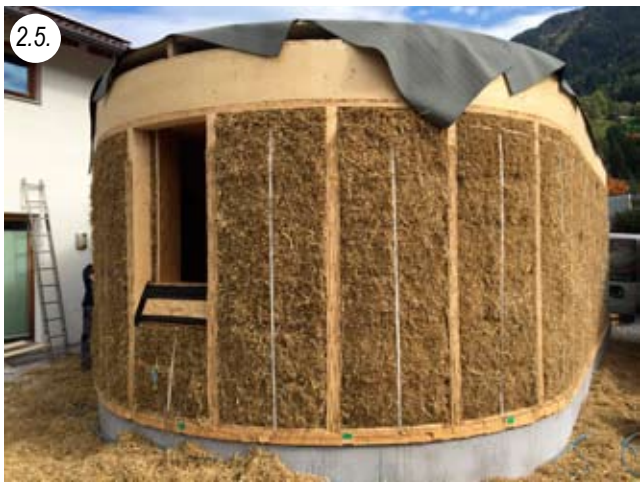
Now the reed mat is stapled onto the wooden surfaces on the front side
