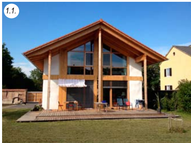
Load-bearing with big bales NUA: 90 m 2 Built: 2010
