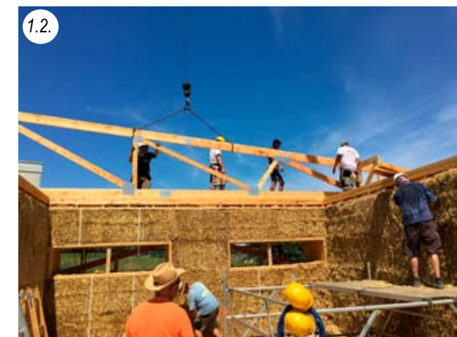
1.2. On the 3rd day the roof truss is mounted
