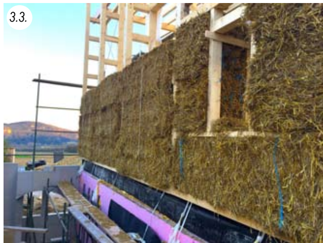
Socket connection with XPS and the threaded straps
