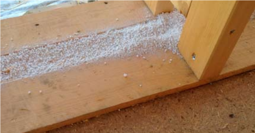
„Condensate pocket“ for any moisture peaks that may occur in the bottom bale of the straw bale wall, space filled with perlite between the floor sills and drainage holes to the outside, below the drip edge. Ready for the first bales.
