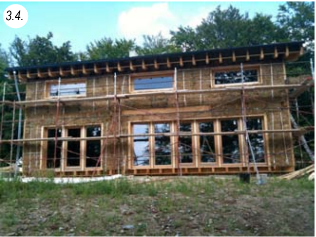
Timber frame with installation level and straw facade in front. Bales doveled to timber wall.
