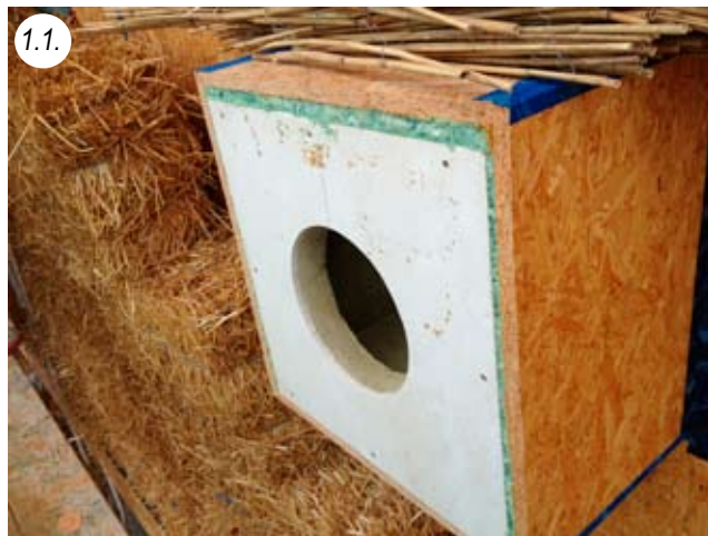
Box for flue gas passage. Inside insulated with rock wool, cover (flush with straw facade) inside and outside made of bromate panels (fire protection panel)
