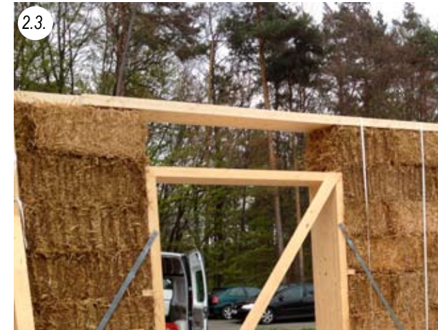
Free space above the windows is only filled towards the end of the settling process
