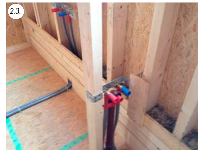
Water connections pre-assembled so that the cavities can be filled with light clay
