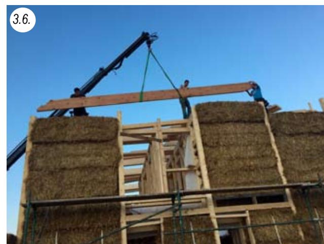
Start of roof assembly
